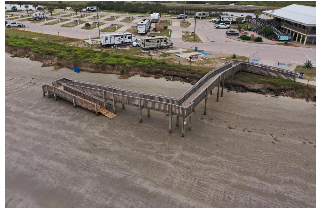
• DELLANERA PARK PEDESTRIAN BRIDGE
