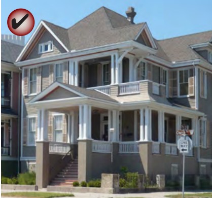
Stucco is often an appropriate foundation enclosure material.
