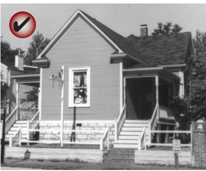
After: Original siding is revealed.
