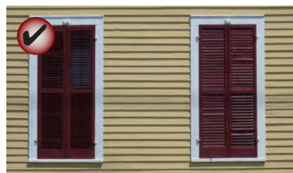
Match the width of new or replacement shutters to the width of the associated window or opening.
