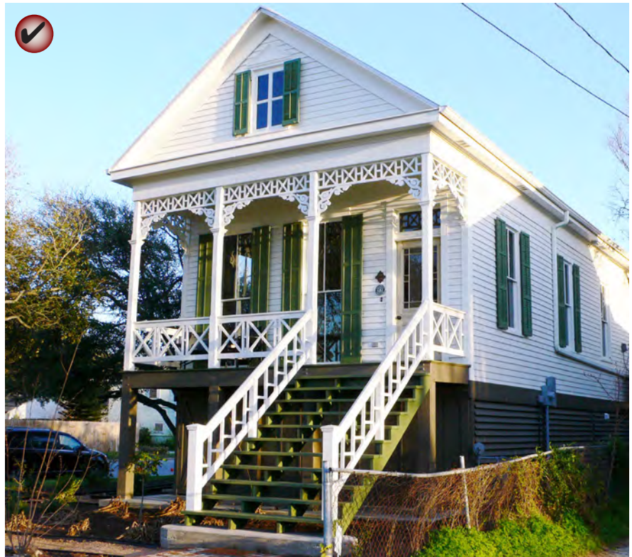
Where space allows, it is appropriate to extend front-facing porch stairs directly towards the street.
