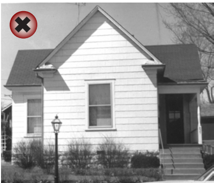
Before: Original siding is obscured.
