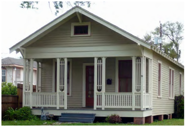
A low-pitched gable roof with wide overhanging eaves and exposed rafter tails are key features of the Craftsman style
