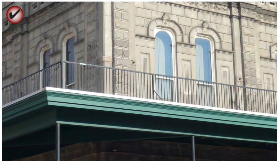
Design a new railing to be as transparent as possible so that it does not obscure the character-defining features of the building.
