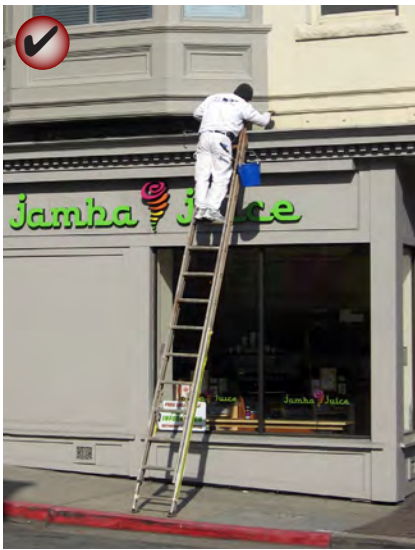
Repair deteriorated building materials.
