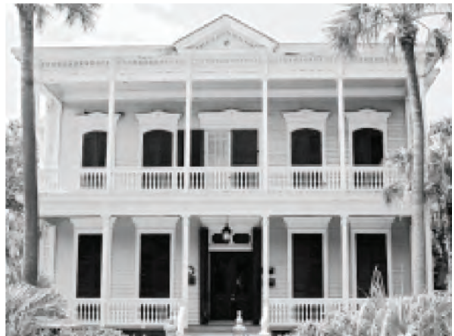
Five-bay Double Gallery Houses are typically larger structures.
